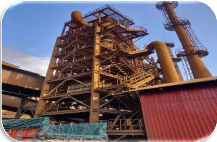
DE system ( Wet Scrubber ) for HSM Silo at SIP.
