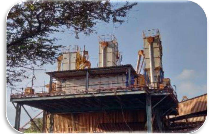
DE system at Various Junction houses of RMHS
