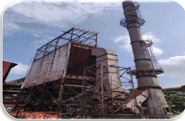
ESP at Discharge end at Pellet
