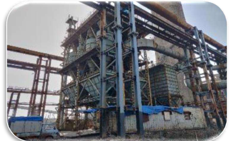
DE system for charging emission at Coke Oven
